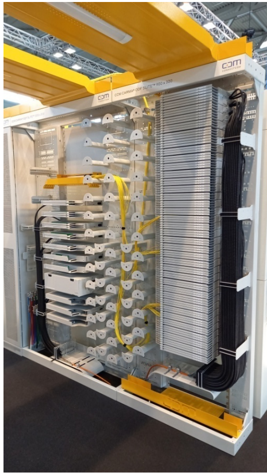
Fig.2. Example of ODF in a Data Center – floor-mounted ODF
