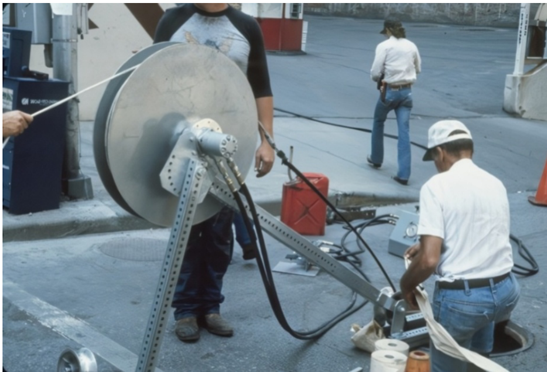
Use of a Cable Pulling Capstan Machine (source: FOA)
