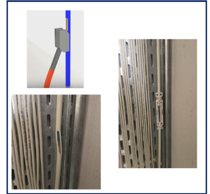
Riser Cable Branching and fixing of the branch unit
