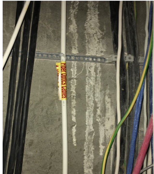
Photos (Above) show FTTH wiring adjacent to MDU power cables; labeling of FTTH riser ducts and separation from power essential.
