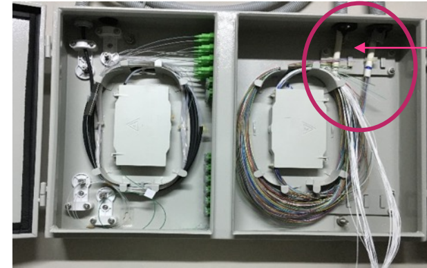
Fibre optics cables protected by ducts & clearly labeled
